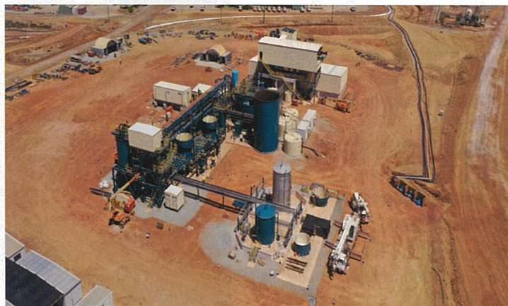
The Wiluna mining concentrator was due to begin commissioning by the end of 2021
