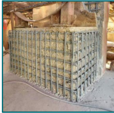
Figure 5: Progression images of concrete remediation work undertaken.
